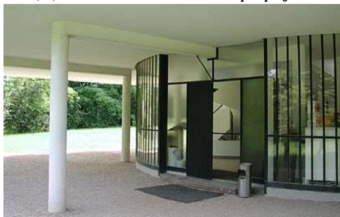
Picture no. (3) Illustrates the idea of a free Facades or open windows- Villa Savoy
